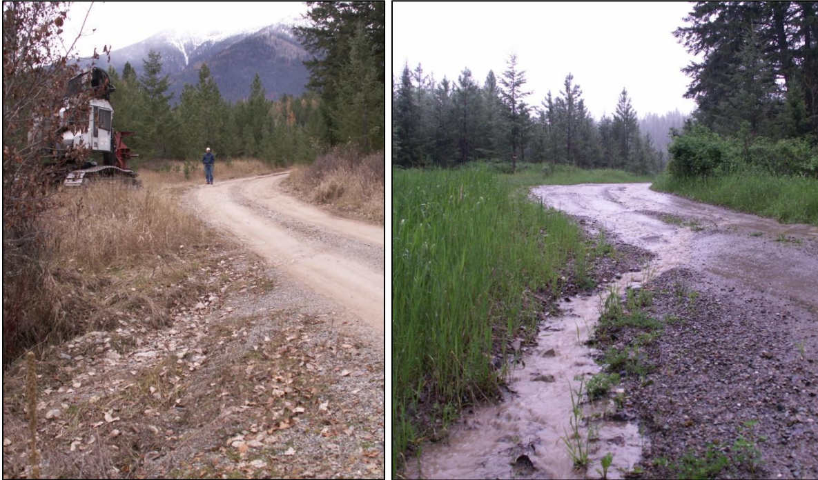
Figure 5-3. An unpaved road sediment source near Sinclair Creek, shown in dry conditions and during a runoff event
