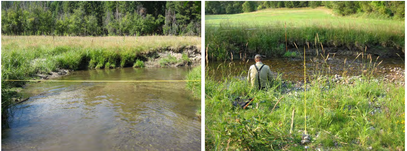
Figure 5-11. Eroding streambanks in the upper (left) and lower (right) portions of Swamp Creek
