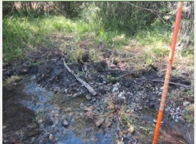
Streambank erosion resulting from livestock access at Gazelle Creek monitoring site GAZL 16-01
