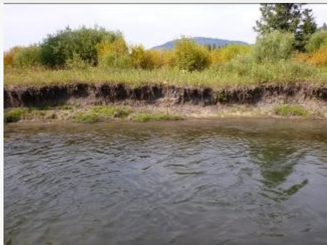
An eroding streambank along the West Fork Madison River at monitoring site WFMA 26-01
