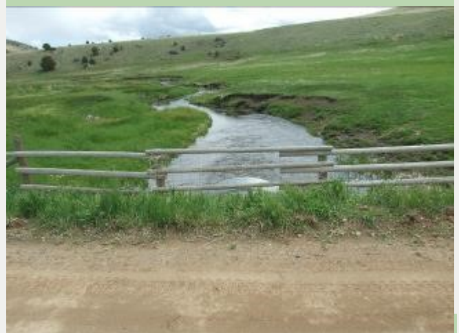
An undersized road culvert and eroding streambanks along Hot Springs Creek
