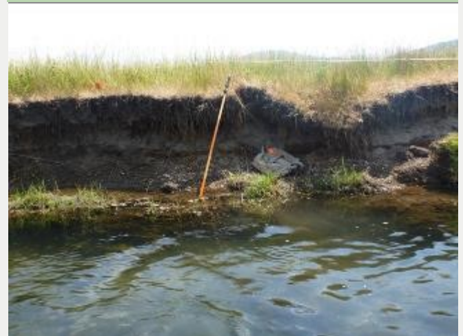
An eroding streambank and poor streamside vegetation at monitoring location CHRR 18-02
