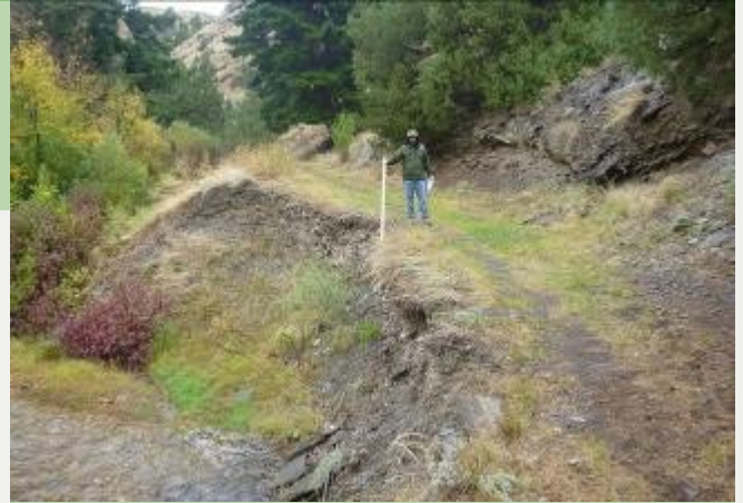
Sediment erosion from an unpaved road along Ruby Creek
