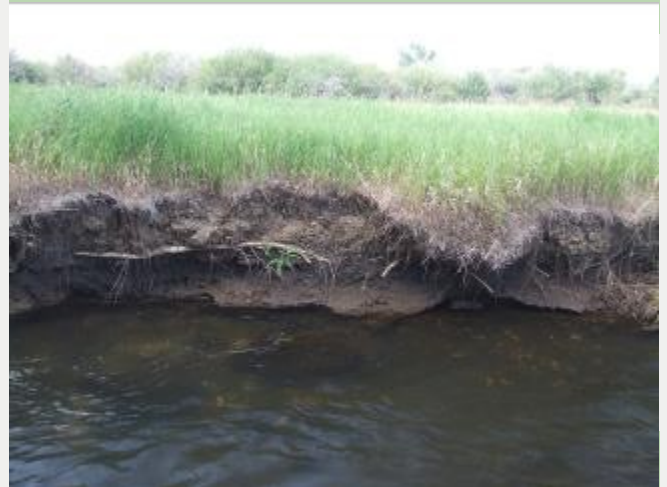
Lack of stabilizing streamside vegetation resulting in an eroding streambank due to livestock grazing
