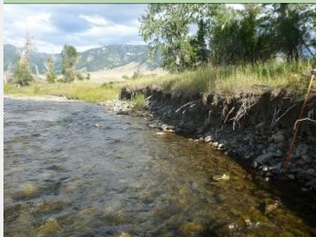
Unhealthy streamside vegetation and an eroding streambank at monitoring site JACK 14-03
