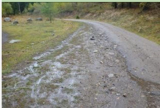
Sediment erosion/runoff from an unpaved road adjacent to South Meadow Creek
