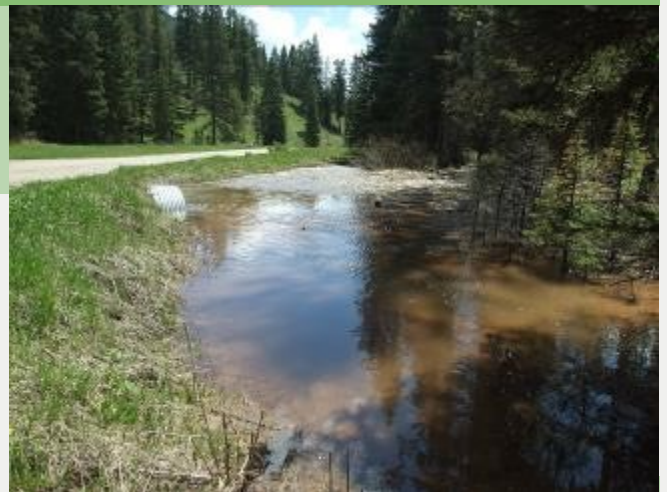
An undersized culvert at a road crossing along Red Canyon Creek
