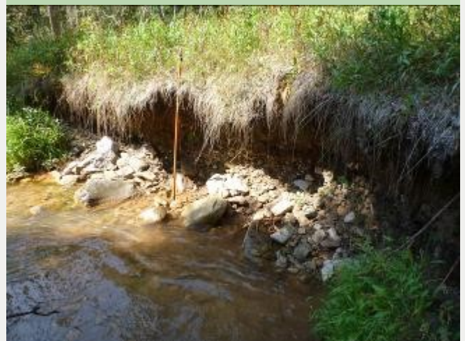
An eroding streambank along Red Canyon Creek
