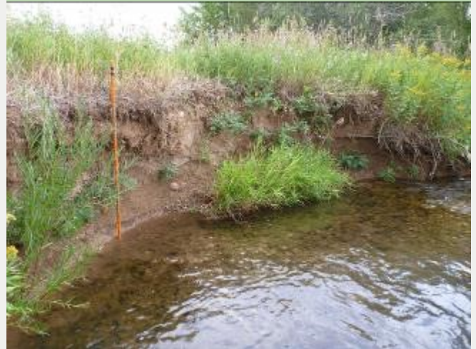
Unhealthy streamside vegetation resulting in an eroding streambank along Ruby Creek
