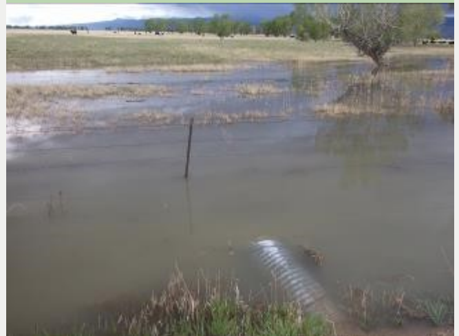
An undersized culvert at a road crossing along Bear Creek
