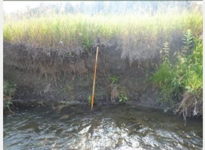
An eroding streambank and poor streamside vegetation conditions on Cherry Creek
