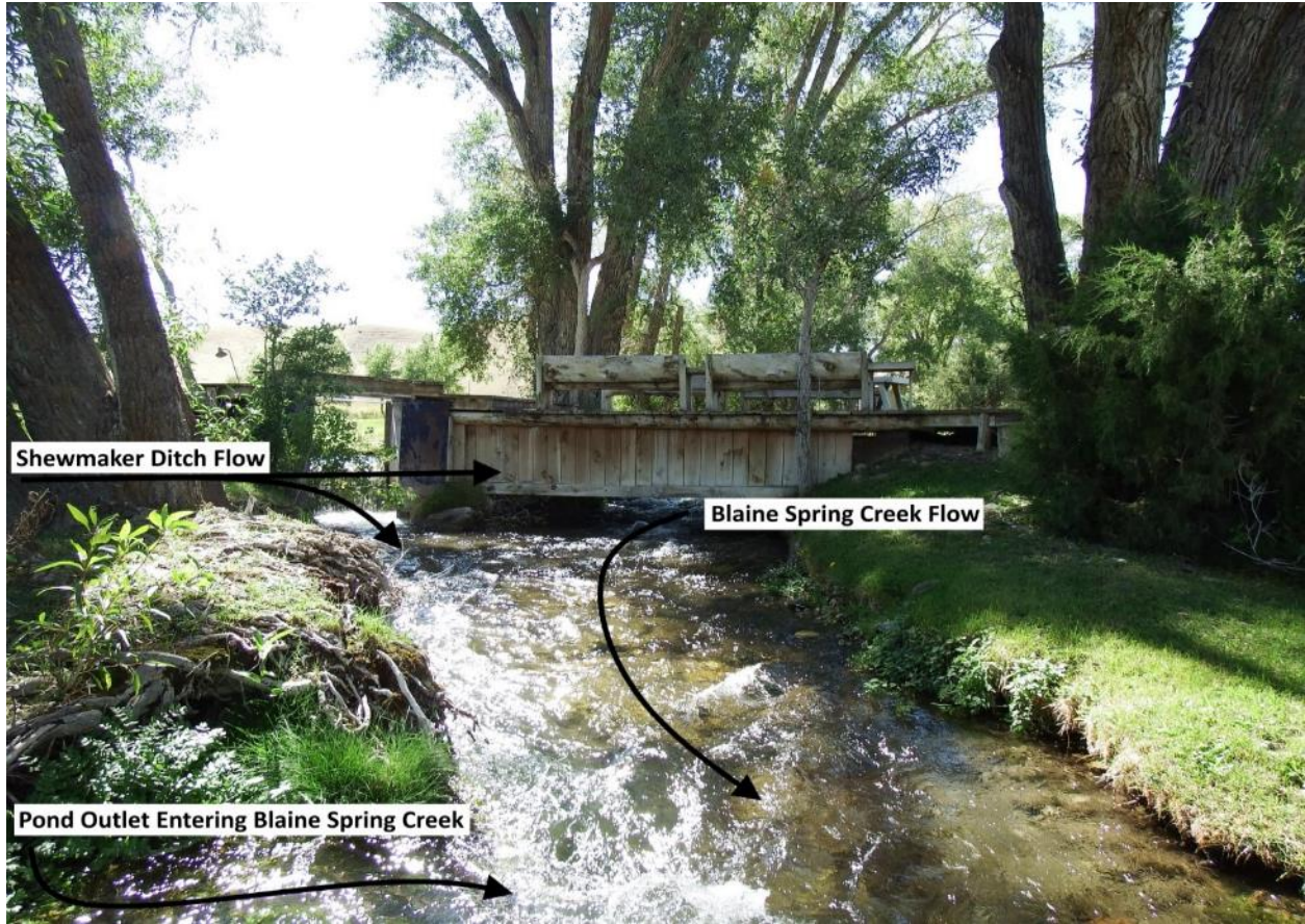
Figure 5-9. Photo showing Shewmaker Ditch crossing Blaine Spring Creek and mixing on the left of the photo
