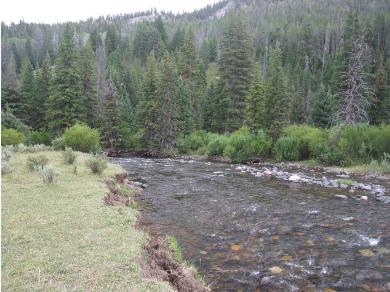
Figure B-9. Eroding streambank at WFMA 25-01
