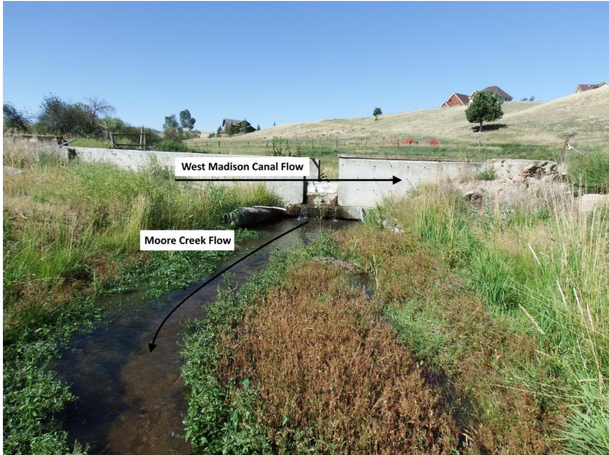
Figure 5-22. Photo showing West Madison Canal crossing Moore Creek and mixing through leaky check-boards in the center of the photo. Headgate releases water into Moore Creek to the left of photo (off photo).
