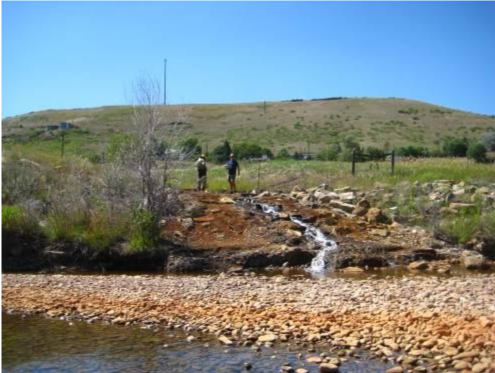
Figure 5-7a. Anaconda Mine Drain discharging to Belt Creek
