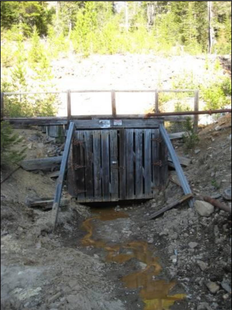
Figure 5-3b. Galena Creek Mine Drain/Adit
