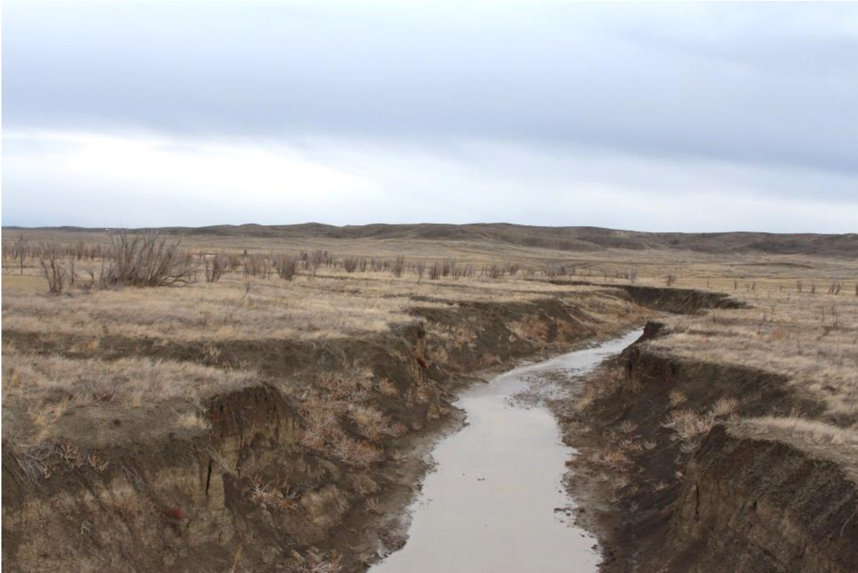
Figure 4 Headcut Through Gutshot Detention Reservoir Bottom
