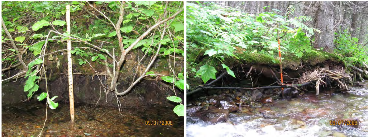
Figure 4-2. Typical streambank conditions in STIL-12 Reach
