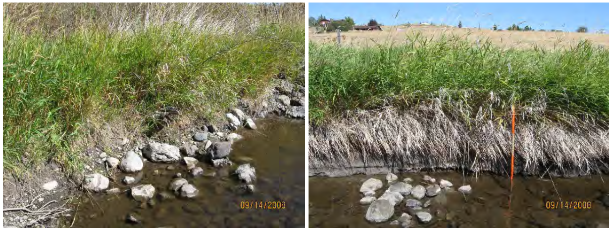
Figure 4-13. Typical streambank conditions in ASHL-29 Reach
