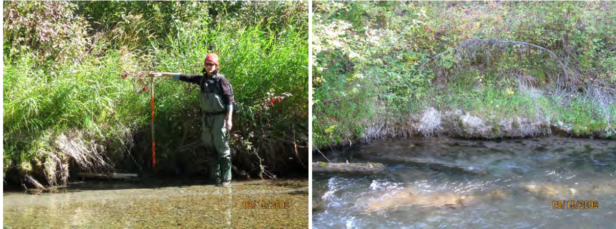
Figure 4-15. Typical streambank conditions in STIL-33 Reach
