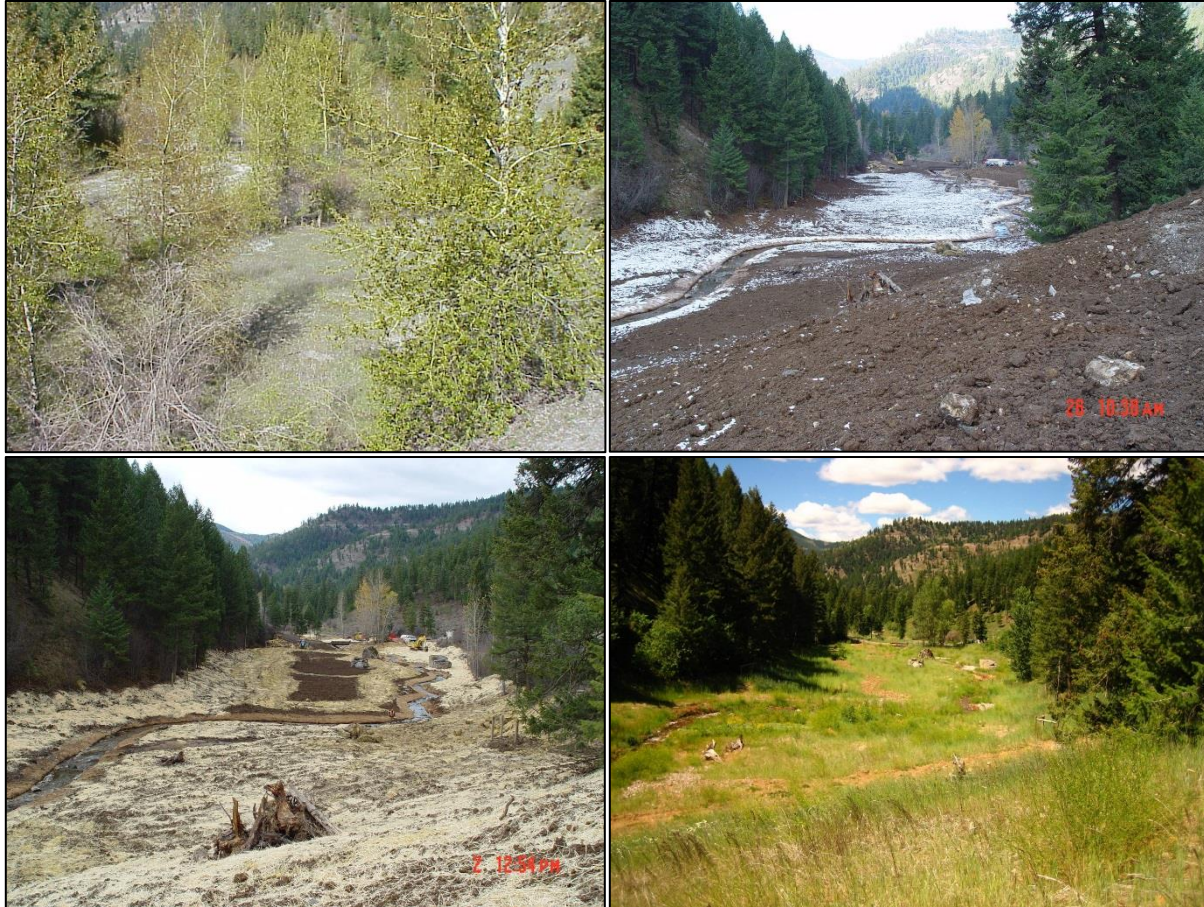
Figure 2 Photos taken from approximately the same point pre-project (top left), after waste removal in 2004 (top right), during seeding and mulching in 2004 (bottom left), and post-project in 2006 (bottom right). Images provided by the Missoula Field Office, BLM.
