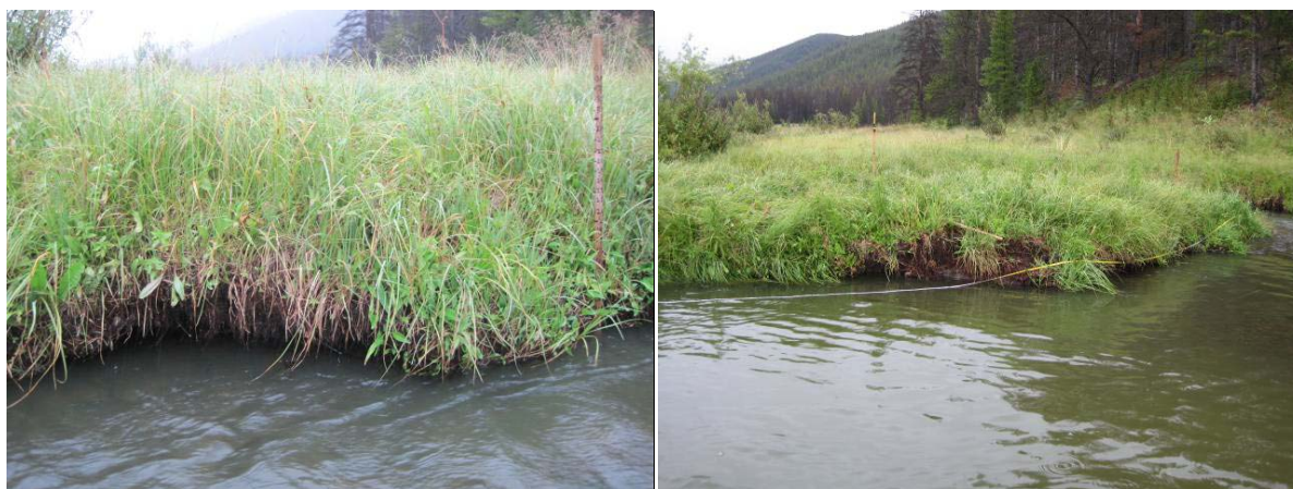
Figure 4-17. Typical eroding streambank conditions in Lowland Creek Reach 08-01.
