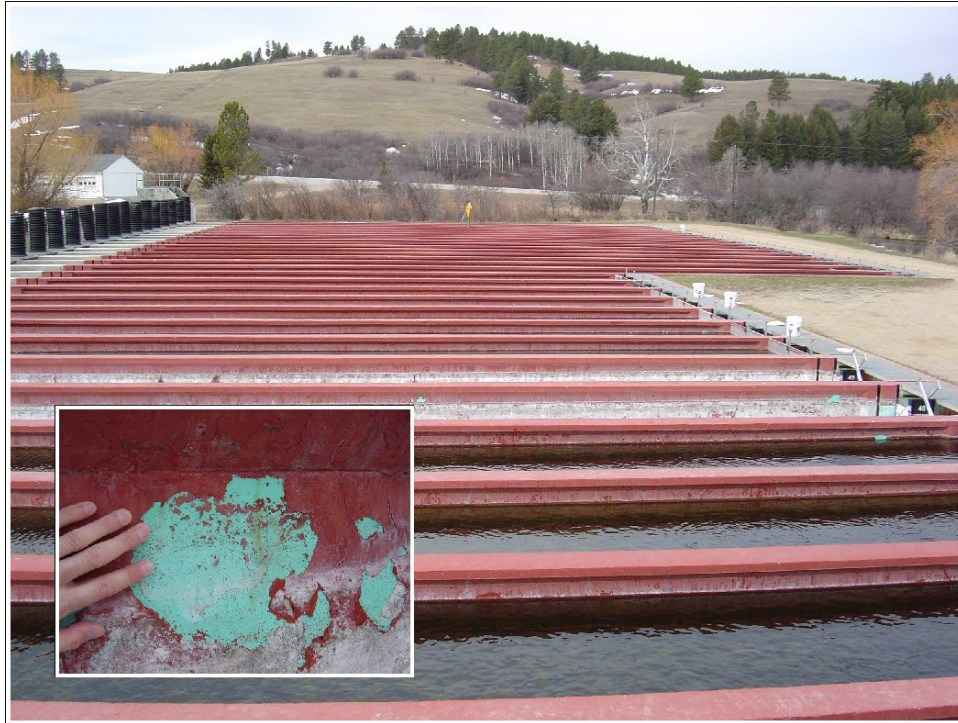
Figure 6-7. Paint containing PCBs at the Big Springs Trout Hatchery – Lower Raceways.
