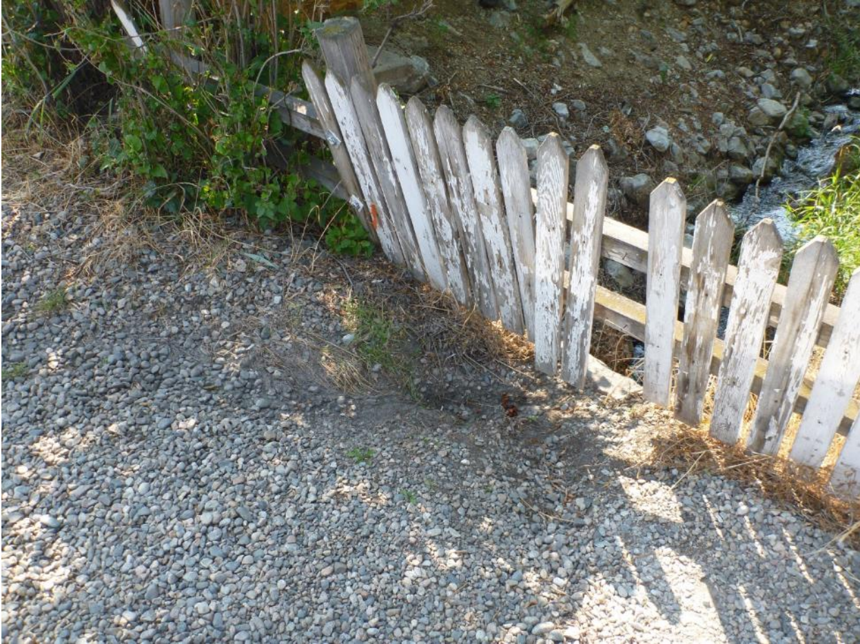
Figure 6-7. Photo showing stormwater discharge point to Moore Creek in the Town of Ennis at the West Main Street crossing (Moore Creek on right)
