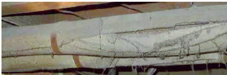
Asbestos insulated pipes typical in older homes.
