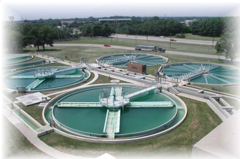
Photo by Montana Water Center – Treatment Plant
