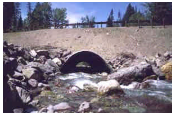
Proper culvert installation keeps water clear.
