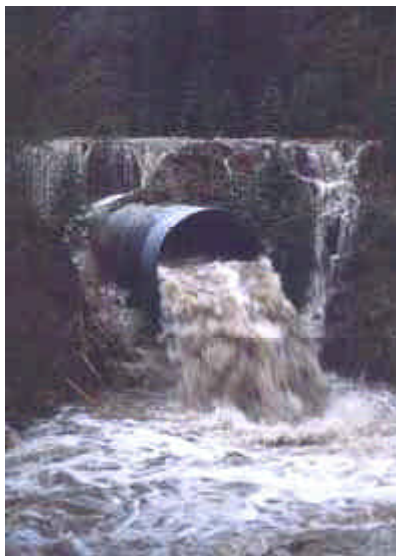
Poor maintenance leads to culvert failure and excess sediment to the stream.
