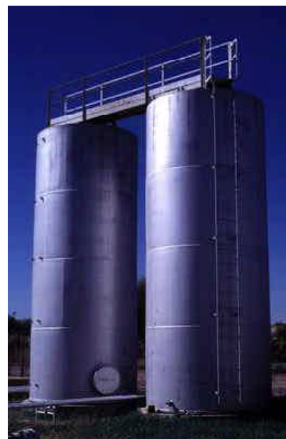
Water Storage Tanks
