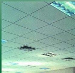
Asbestos-containing ceiling tiles will not be labeled or marked. These tiles cannot be differentiated from other tile by visual means - they must be analyzed by a laboratory test.
