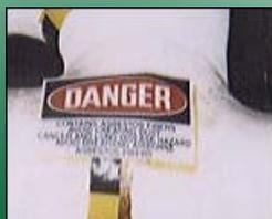
Pipe and boiler insulation that contains asbestos should be labeled with identifying stickers and placards.
