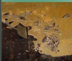
Asbestos is most hazardous when it is **friable**. The term "friable" means that the asbestos is easily crumbled by hand, releasing fibers into the air. Sprayed on asbestos insulation is highly friable. Asbestos floor tile is not.
