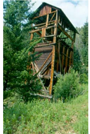
Ore Loadout Tower
