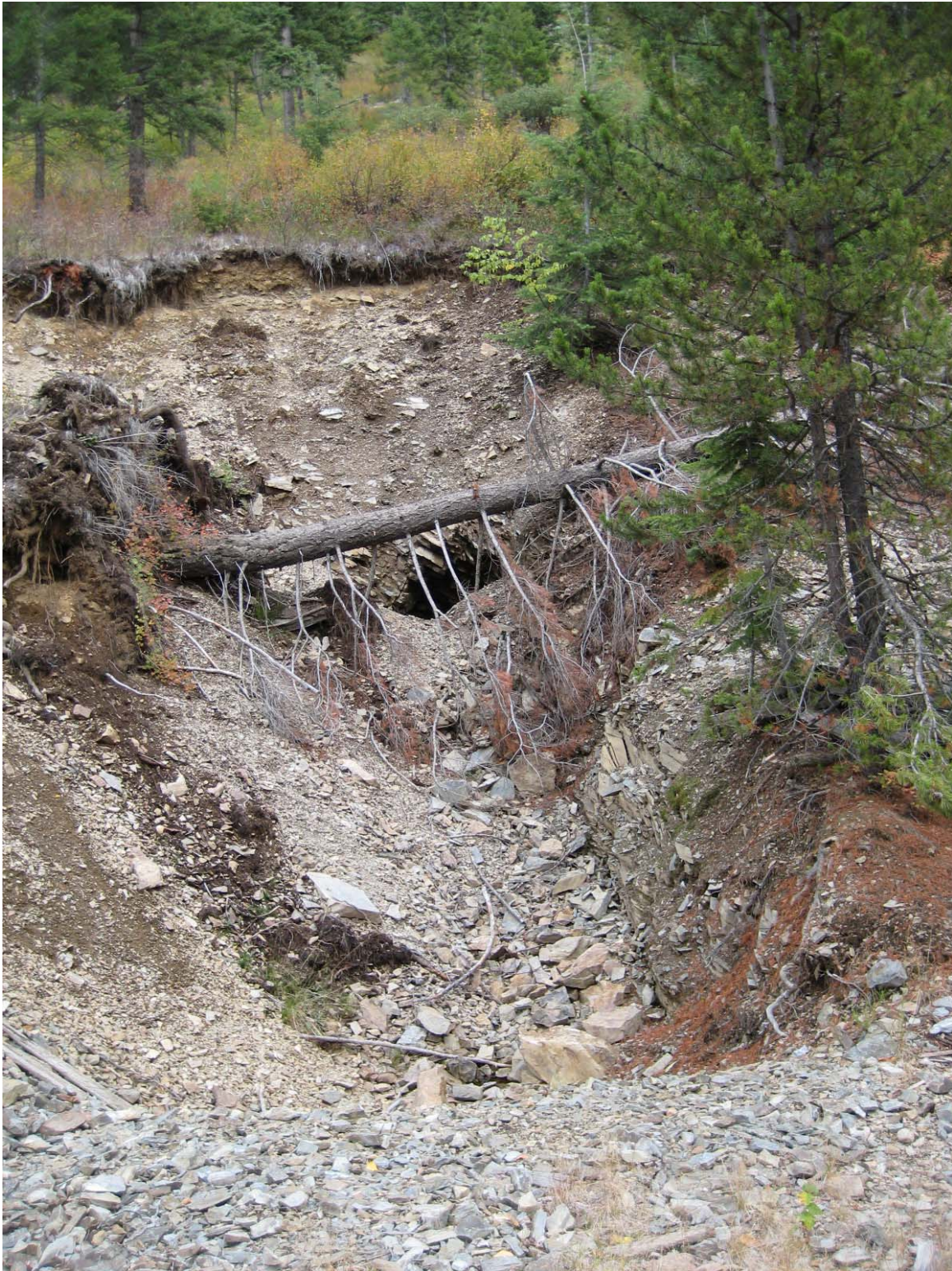
Figure C-4. Adit at the lower waste rock dump.
