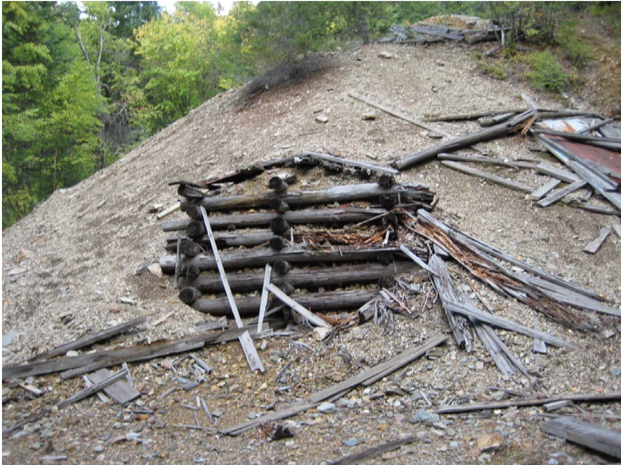
Figure C-6. Lower waste rock dump with the ore loading chute.
