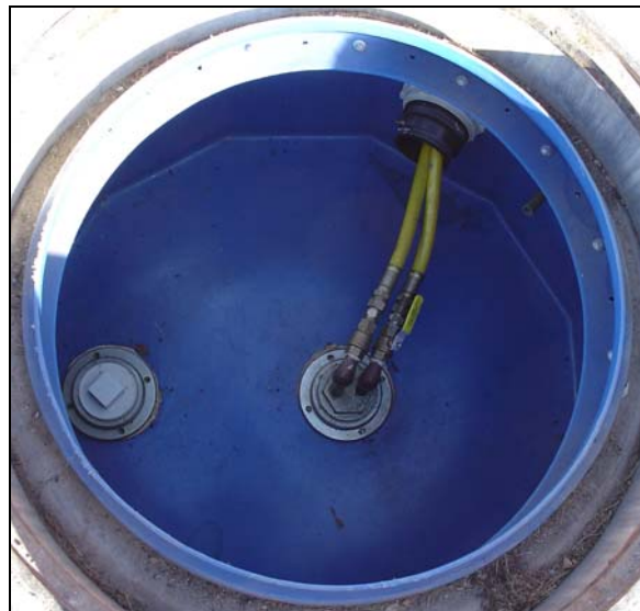
Sample Sump of a Suction system (U.S. Suction)
