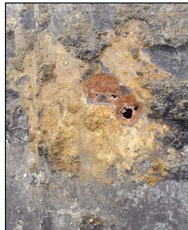
Hole in a metal tank from corrosion
