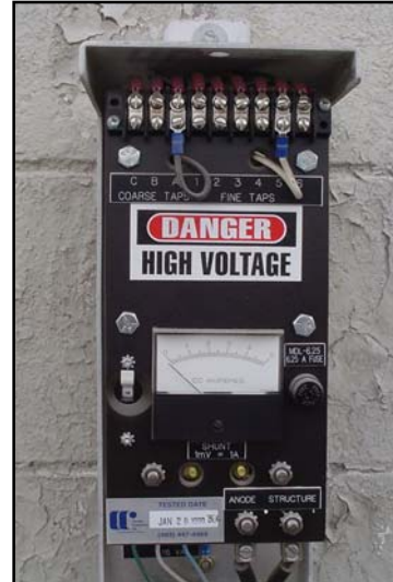
Rectifier Box for An Impressed Current System
