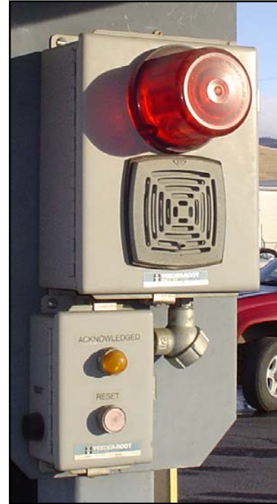
Sample Overfill Alarm
