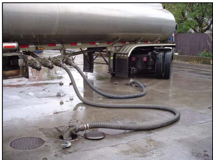
Fuel Drop Into An UST
