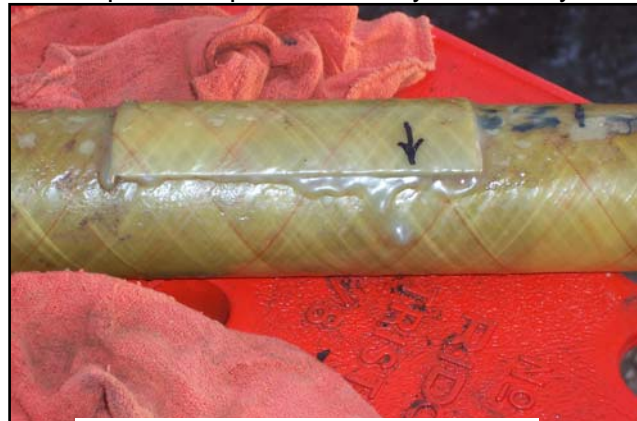
Repaired FRP Piping
