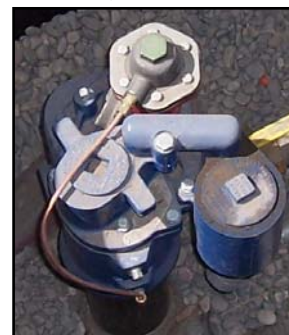
LLD Installed on a Submersible Turbine Pump
