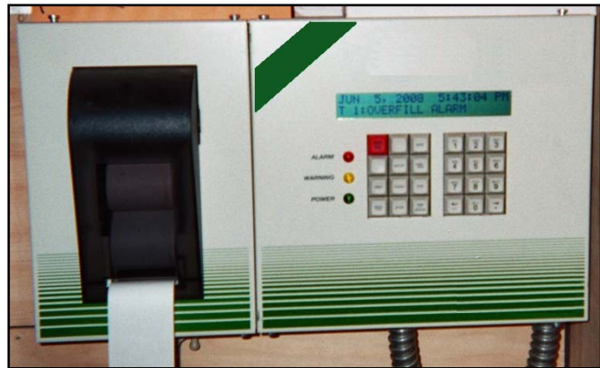
Sample ATG in Alarm
