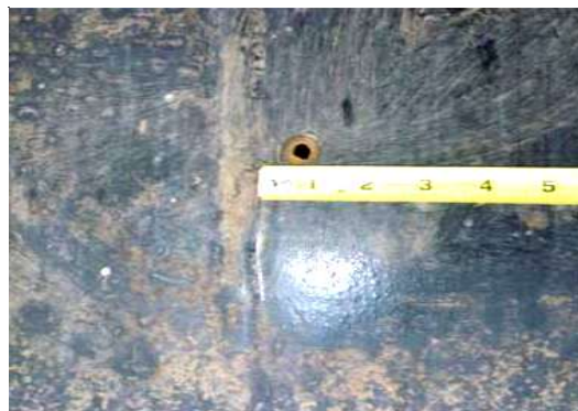
Outside view of a hole in a leaking steel UST
