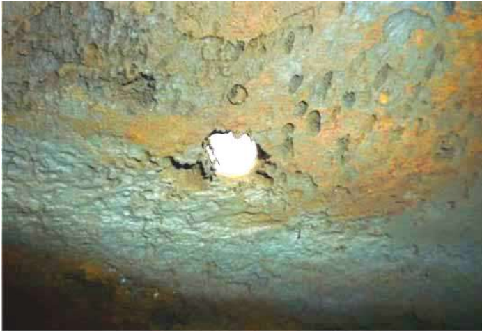
Inside view of the same hole in the same leaking UST
