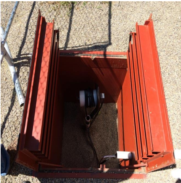
Reel Assembly in protective vault
