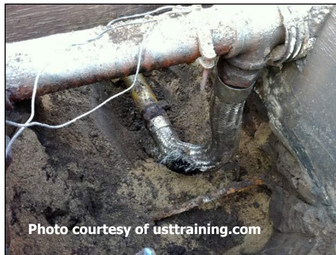
FIGURE 2: A failed flex connector.
