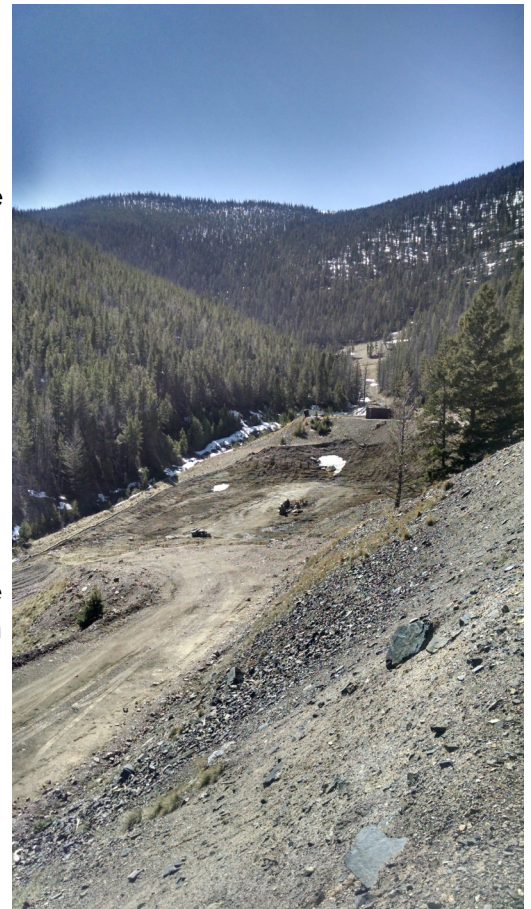
Looking up Mike Horse Creek at the excavation of the old Mike Horse Repository.
