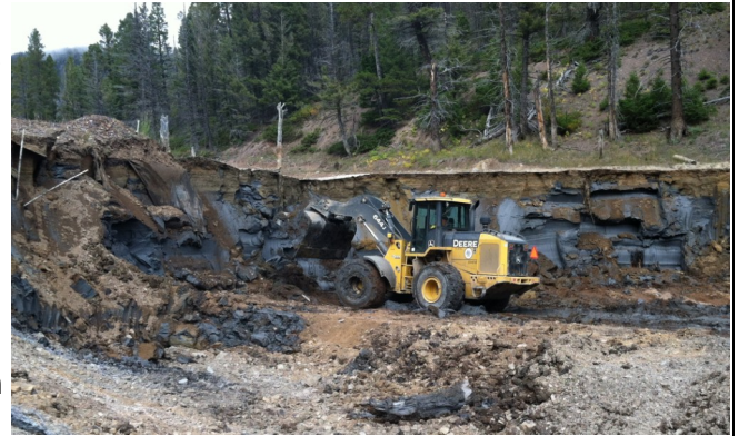
Excavating tailings behind the Mike Horse dam.
