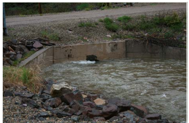
Culvert underwater at water treatment plant, 6-7-11
