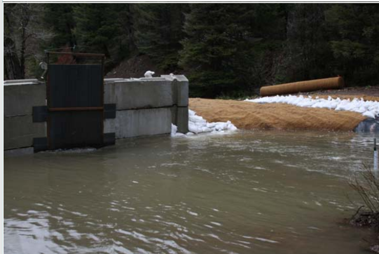
Left photo: spillway next to headgate shored up with sandbags
