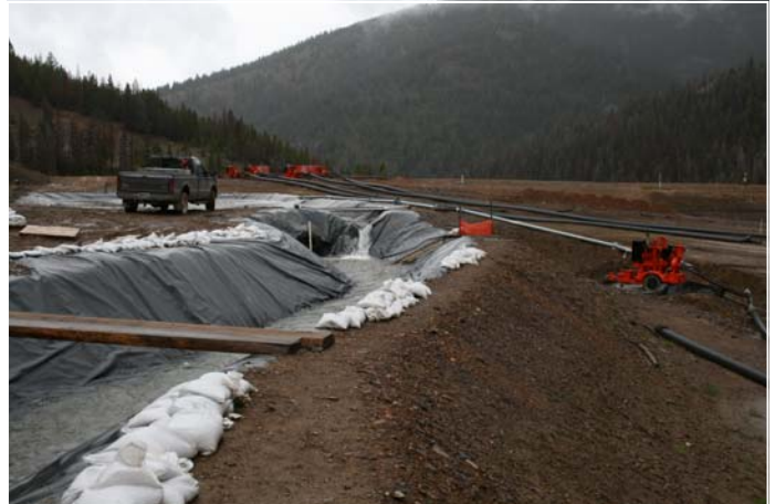
Sandbags along diversion ditch, pumps and pipes. Impoundment off to the right
