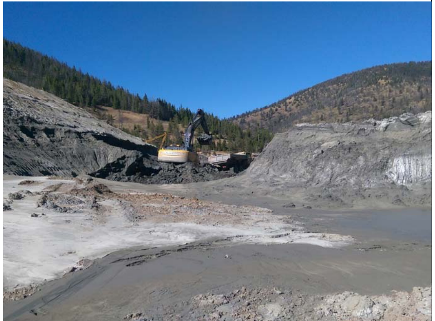
Above: The moment that contractors broke through the "dam."
