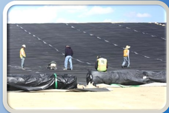
Liner being laid down during new landfill construction.
