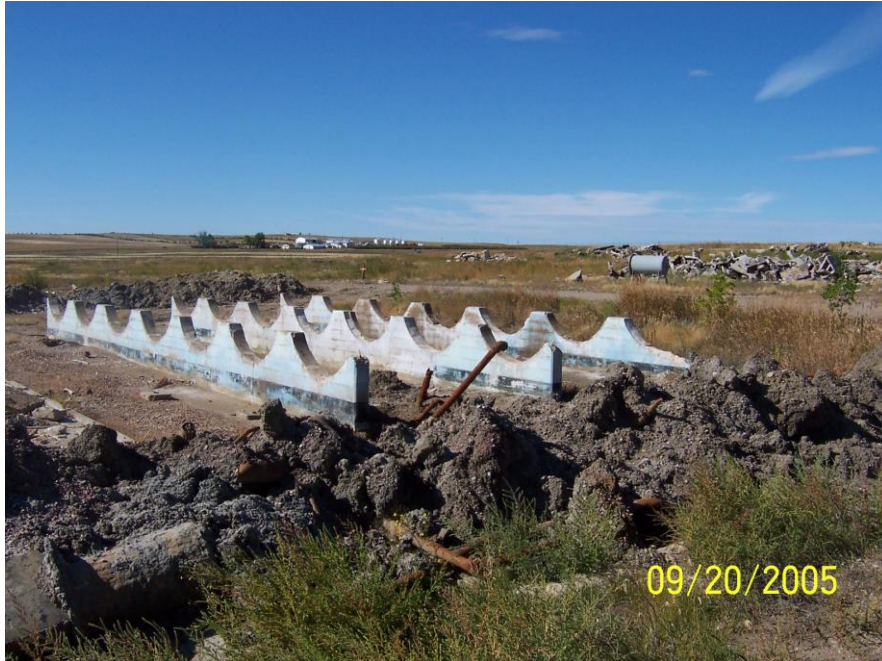
Process Area of the Former Flying J Refinery
