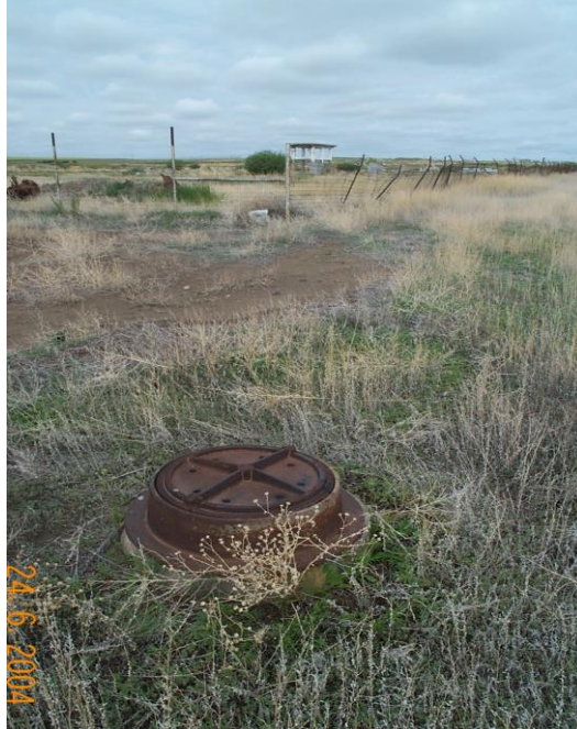
Part of the Refinery wastewater system
