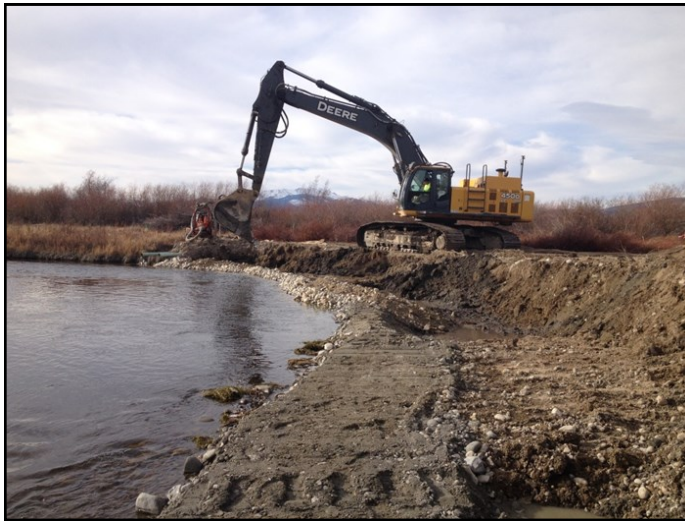
During excavation, the banks may be steepened, the floodplain may be rough and sloughing can be dangerous to untrained personnel.
