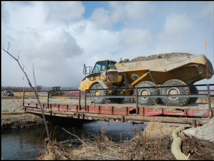
Temporary bridges crossing the Clark Fork River and temporary dams are impassable to floaters. Portage would be extremely dangerous and will not be allowed due to a National Park Service Floodplain Closure.
