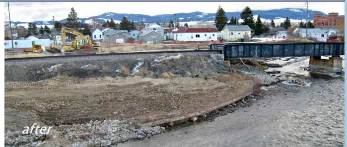
Completed streambank and crib wall upstream of the railroad trestle.
