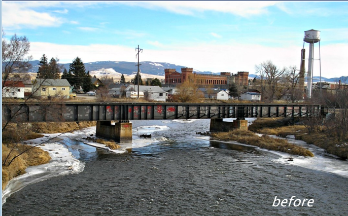
Trestle area before construction
