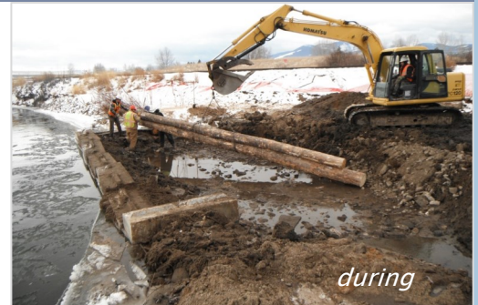
Construction of the crib wall to prevent erosion of the railroad grade into the river.
