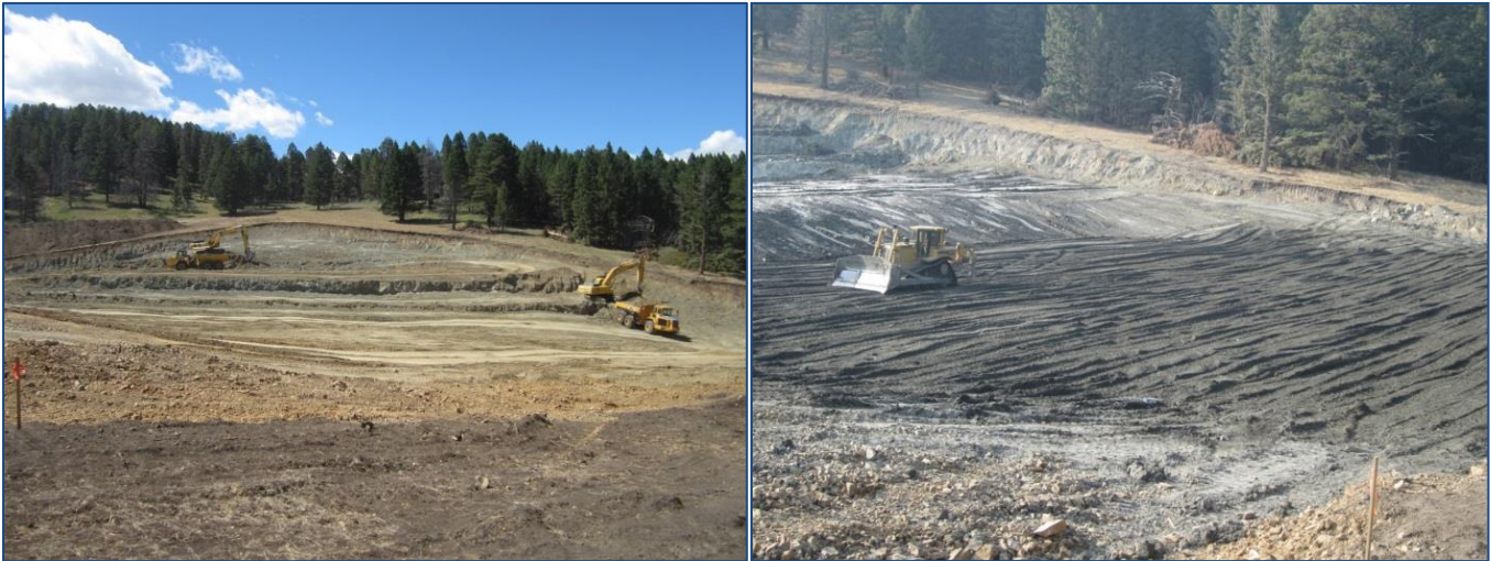
Figure 5 Excavating and Placing Waste in a Repository
