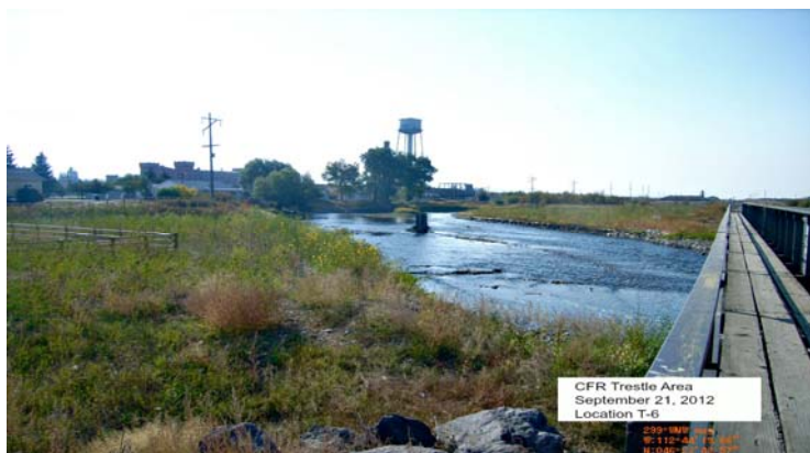
The Trestle Post— Construction September 2012
