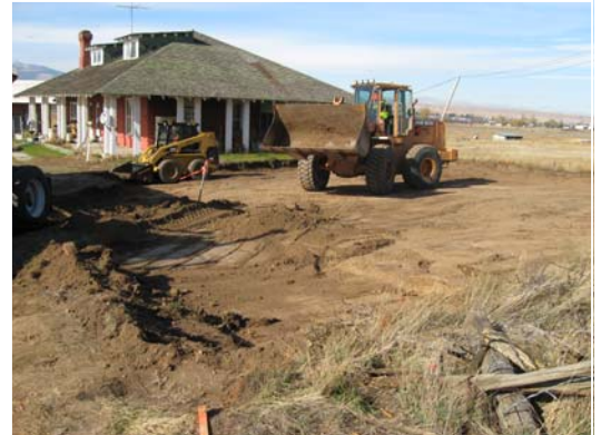
Removing contaminated soil from residential yard, fall 2010
