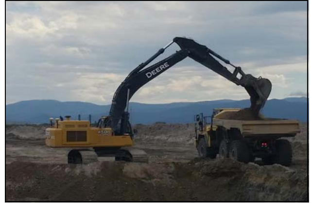
Internal haul roads were constructed with gravel from an onsite source in preparation for hauling of contaminated materials.
