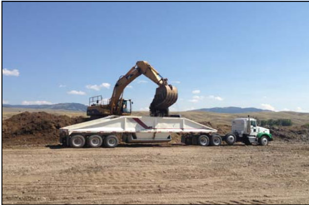
Trucks are loaded onsite with contaminated materials for transport to the BP/ARCO Waste Management Area.
