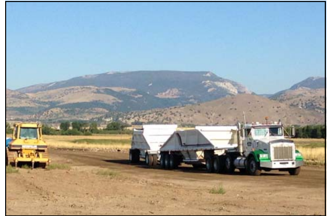
Trucks deposit contaminated materials in the repository within the Waste Management area..
