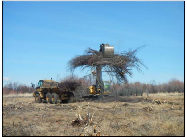
Woody material (decaying willows) was removed and stockpiled for eventual placement in the floodplain to create roughness and natural seed bed niches.
