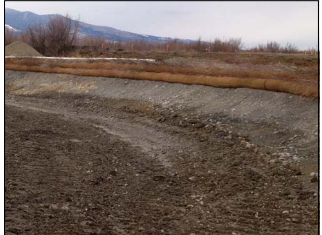
Double vegetated soil lifts were constructed to form the new channel banks.
