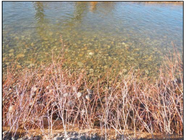
Clean channel bed rock of appropriate native material size was used to rebuild the streambed.
