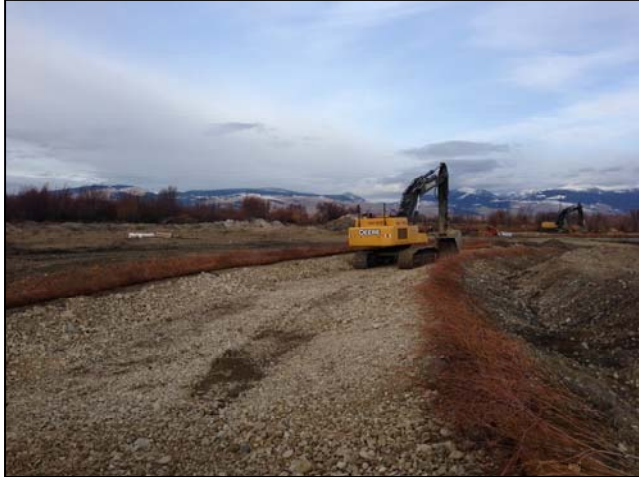
The excavator operator works to shape the streambed materials in the rebuilt Clark Fork River channel.
