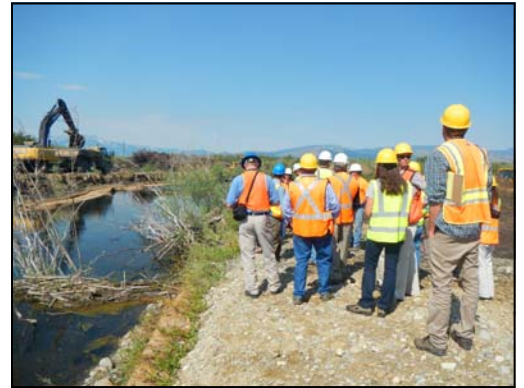
The group looks on as a streambank is being reconstructed by Helena Sand and Gravel backhoe operator Myron Belgarde and the Stream Team.
