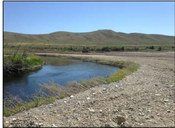
The same river bank after cleanup. The contamination was removed, the floodplain was lowered and the decadent and decaying willows were replaced with bio engineered streambanks and native vegetation.
