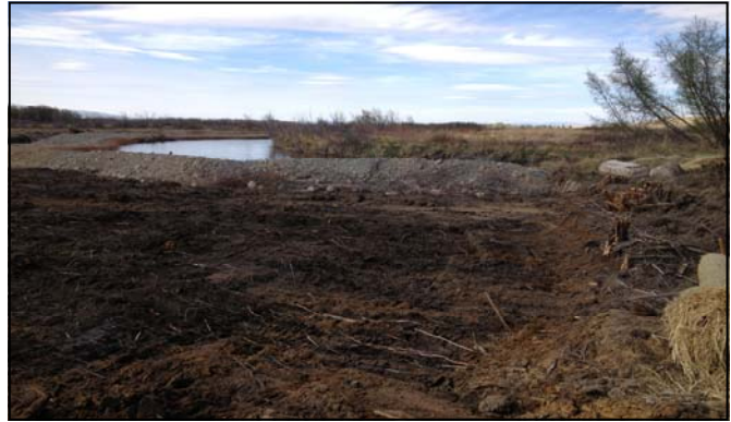
Berming along the river in preparation for high water. Tailings were previously removed from the floodplain—May 2013
