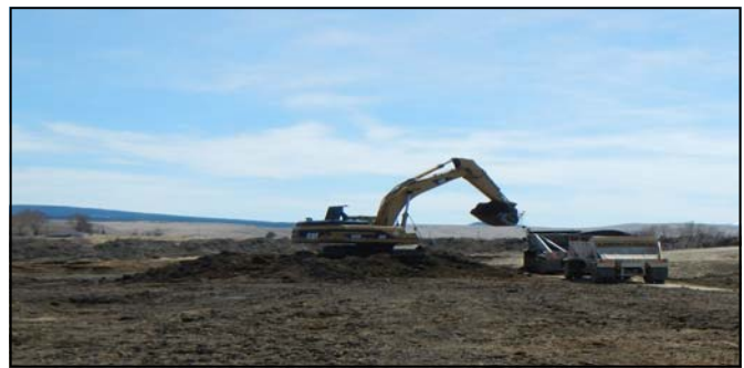
Contaminated Material being excavated from the floodplain and being transported to the BP ARCO Waste Management Area—May 2013
