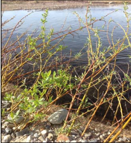
Recently reconstructed stream-bank, using live willow cutting. Willow were collected from locations in the Upper Clark Fork Basin—May 2013
