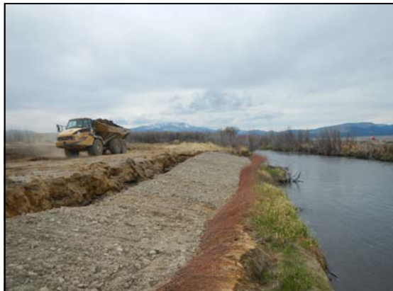
Preserved vegetation with a brush trench streambank treatment—May 2013
