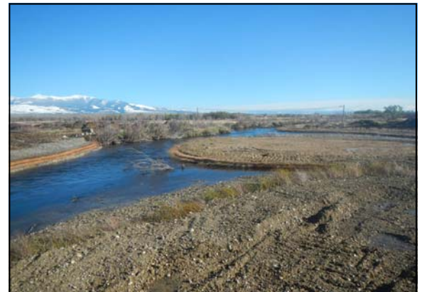
Stabilized streambank on both sides of the river—May 2013
