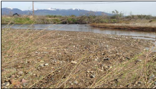
Recently reconstructed point bar (front) and double vegetation soil lift (back) - May 2013
