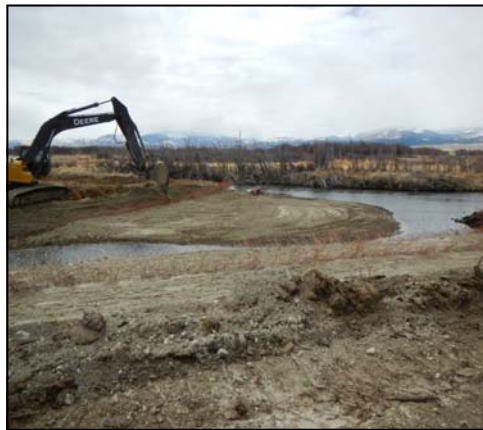
Tailings removal and streambank stabilization— April 2013
