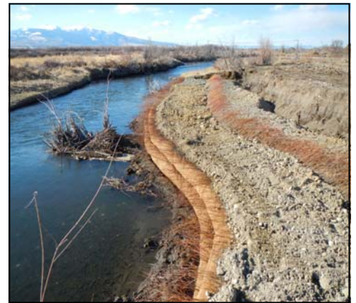
Stabilized streambank - April 2013
