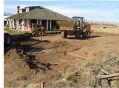
Removing contaminated soil from residential yard, fall 2010
