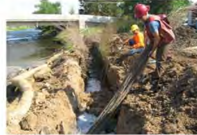
Removing contaminated soil from residential yard and rebuilding stream banks, summer 2011
