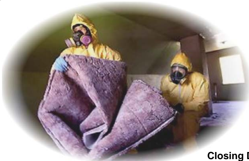
Removal of meth-contaminated carpet
