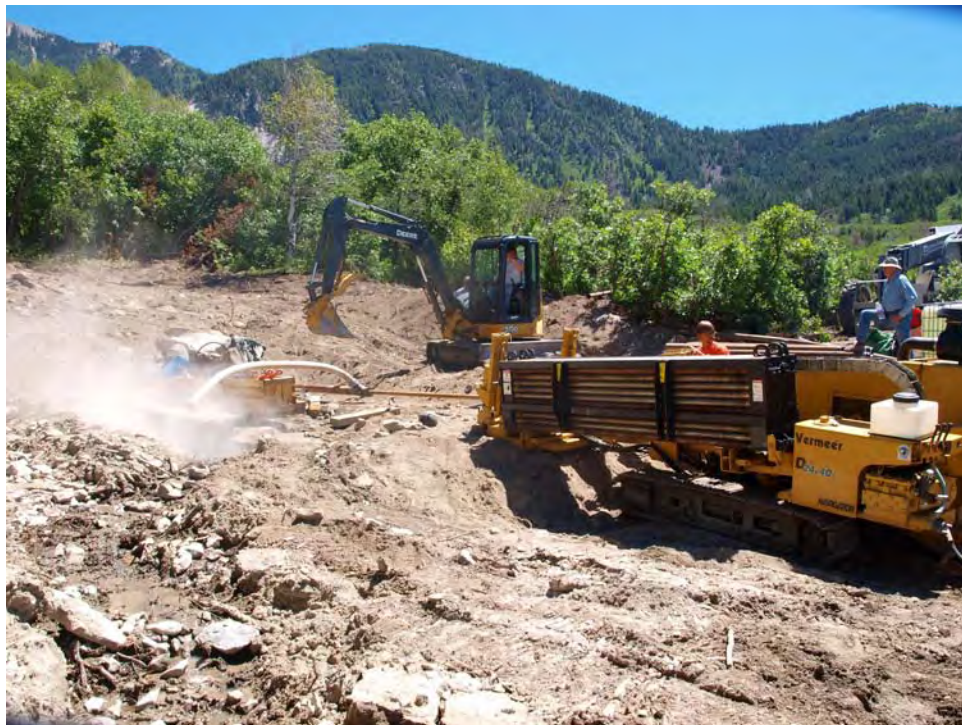
Horizontal Drill Rig on Drill Pad
