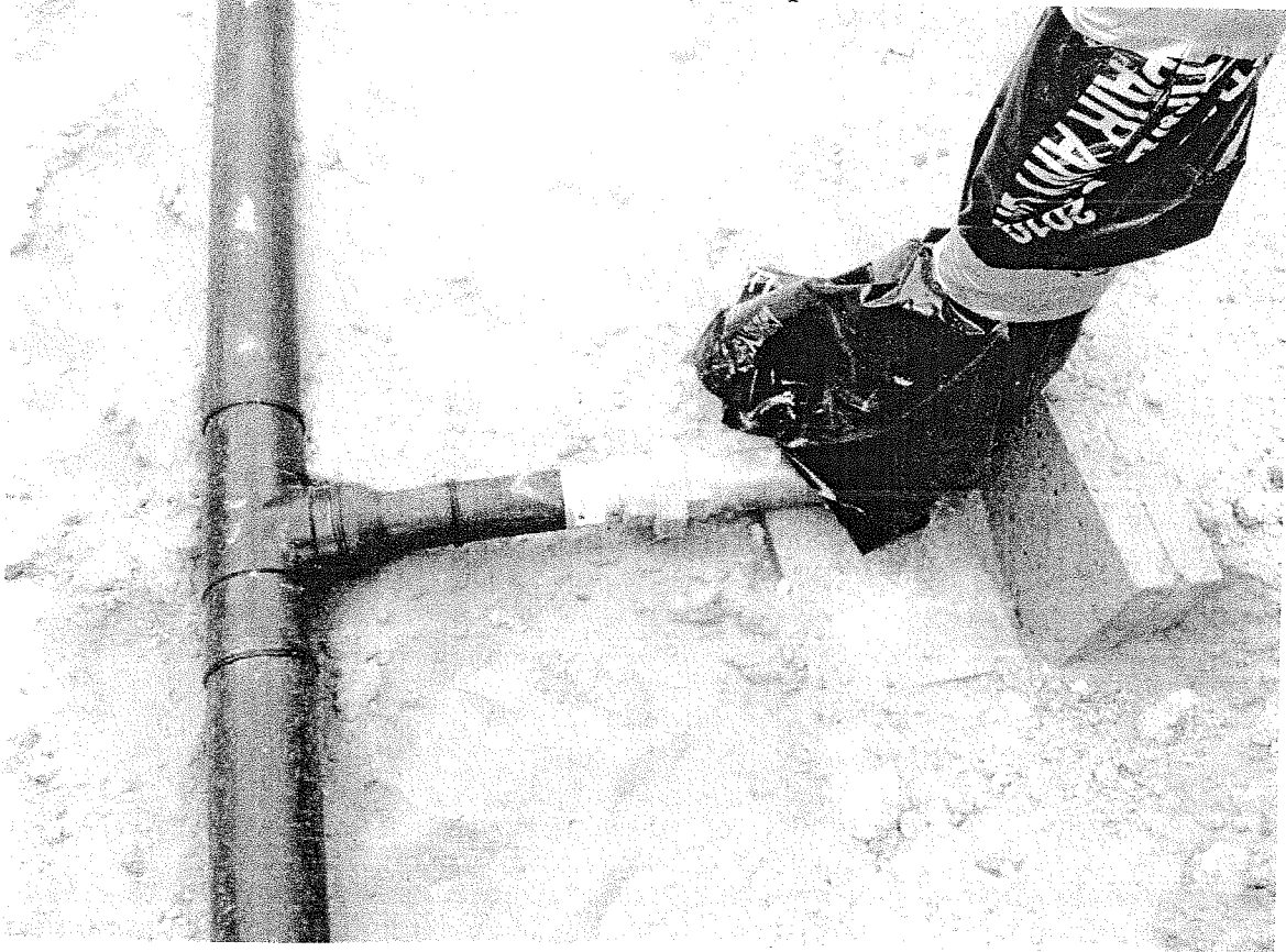
Photo 5: Connection of 3" HDPE line to new 2" diameter post hydrant. Note heat welded 3" tee and 3" to 2" concentric reducer. Also note brass union and type K copper to hydrant. Brass union was wrapped in 6 mil poly after photo.
