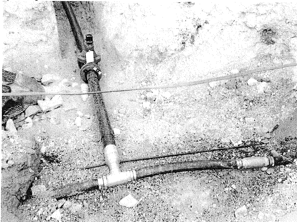
Photo 4: Connection of new 3" HDPE line to existing 2" HDPE line; note 3" gate valve, stainless tee and reducer, and brass check valve. Gate and check valves were wrapped in 6 mil poly after photo.
