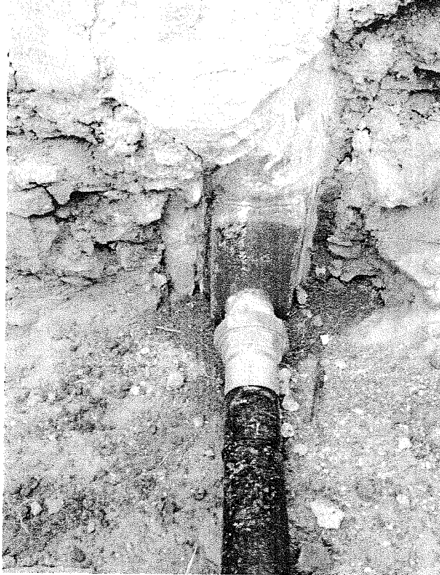
Photo 4: Connection of new 3" HDPE line to existing 2" HDPE line; note 3" gate valve, stainless tee and reducer, and brass check valve. Gate and check valves were wrapped in 6 mil poly after photo.
