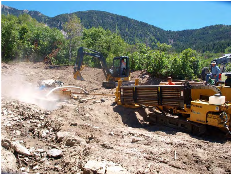
Horizontal Drill Rig on Drill Pad
