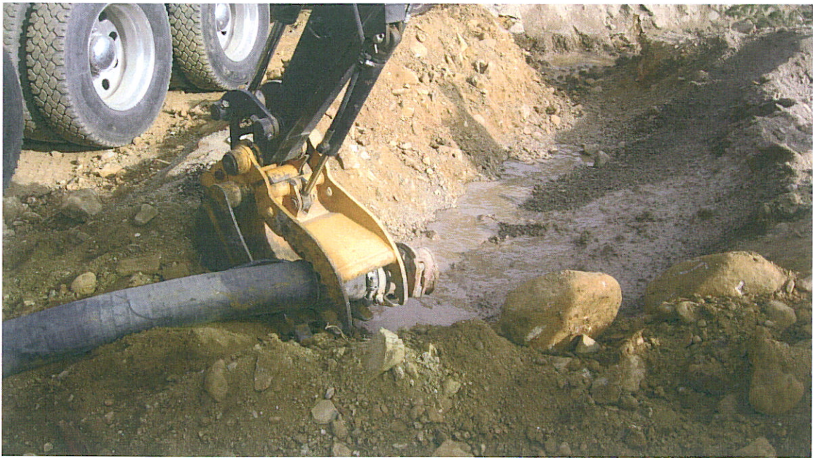
Controlling discharge line with excavator bucket at well C3-6
