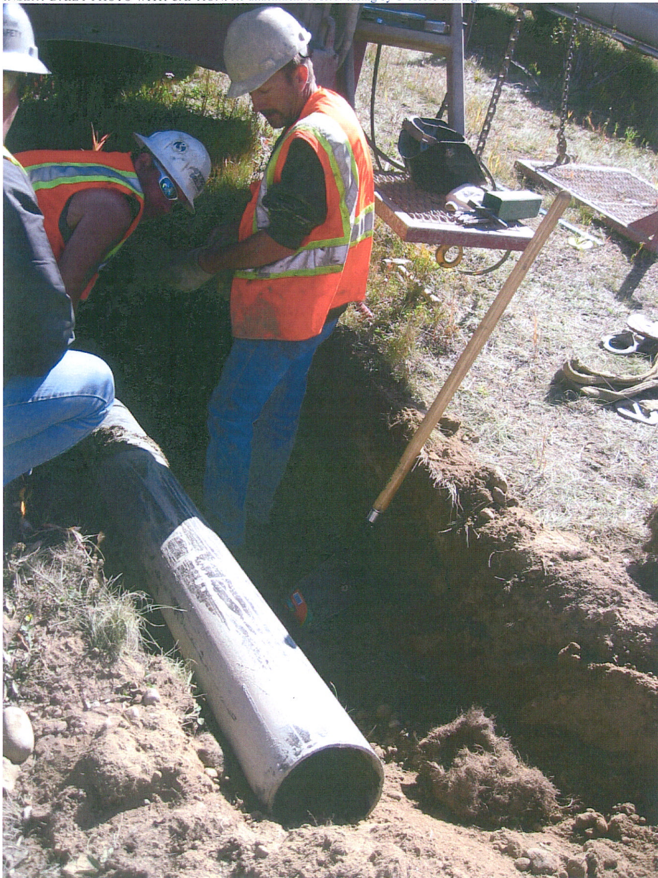
INSERT DAILY PHOTO WITH CAPTION: Re-attachment of steel casing by O'Keefe drilling.
