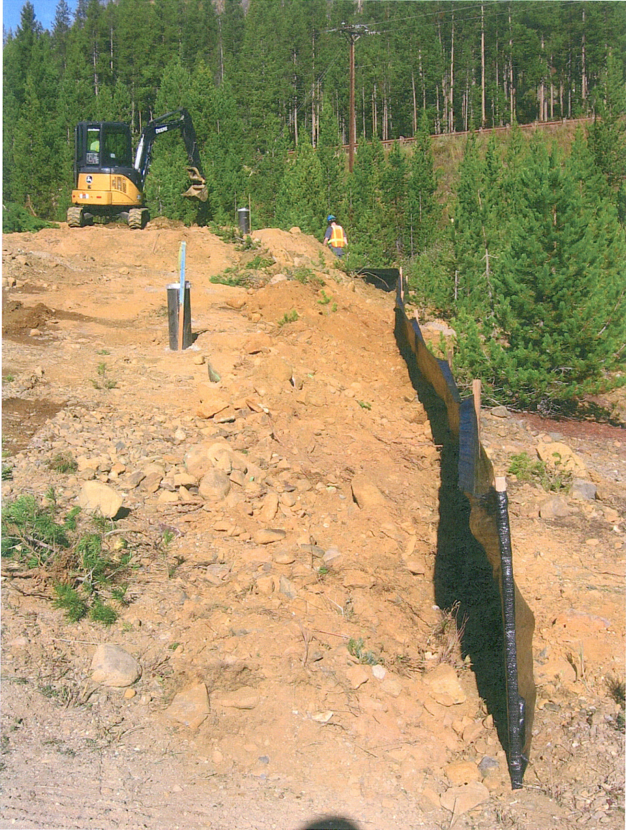
INSERT DAILY PHOTO WITH CAPTION: Installation of silt fence by Bear Claw Construction.
