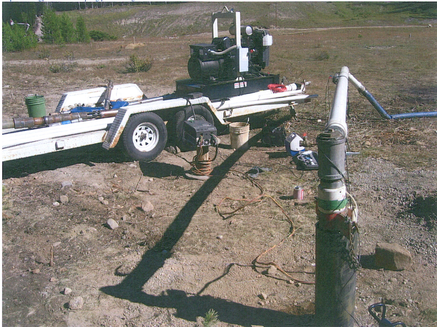
INSERT DAILY PHOTO WITH CAPTION: Pumping of C3-1 by Chamberlain pump with 3 phase setup and 4-inch discharge line. Pumping rate at time of photo: 80 gpm. Note sampling port and digital flow meter.
