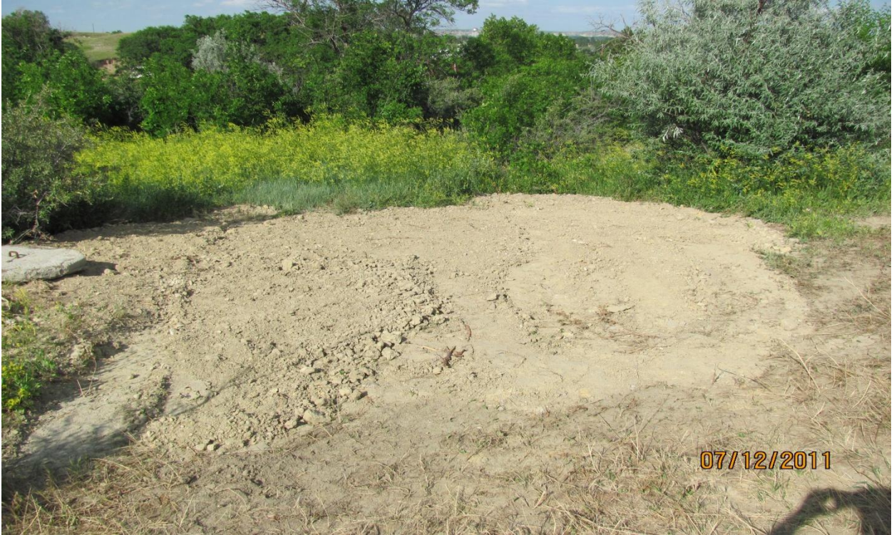
Completed subsidence backfill
