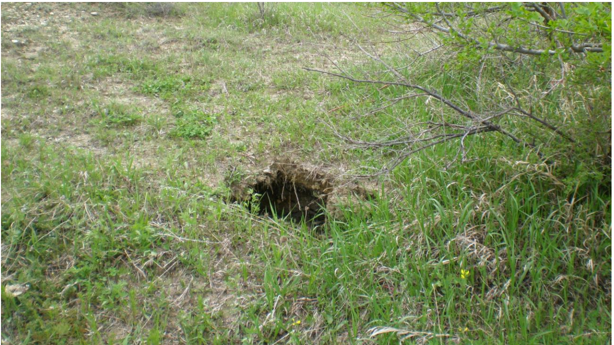
Additional Subsidence on Daniels property
