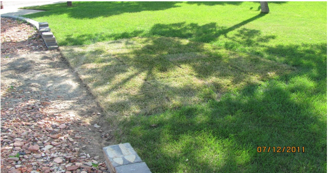
Completed Subsidence backfill adjacent to Gardner Residence.
