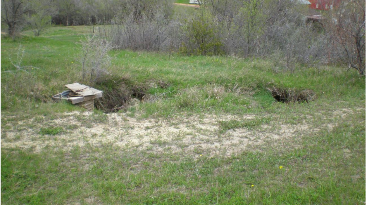
Daniels Well Collapsed into subsidence features
