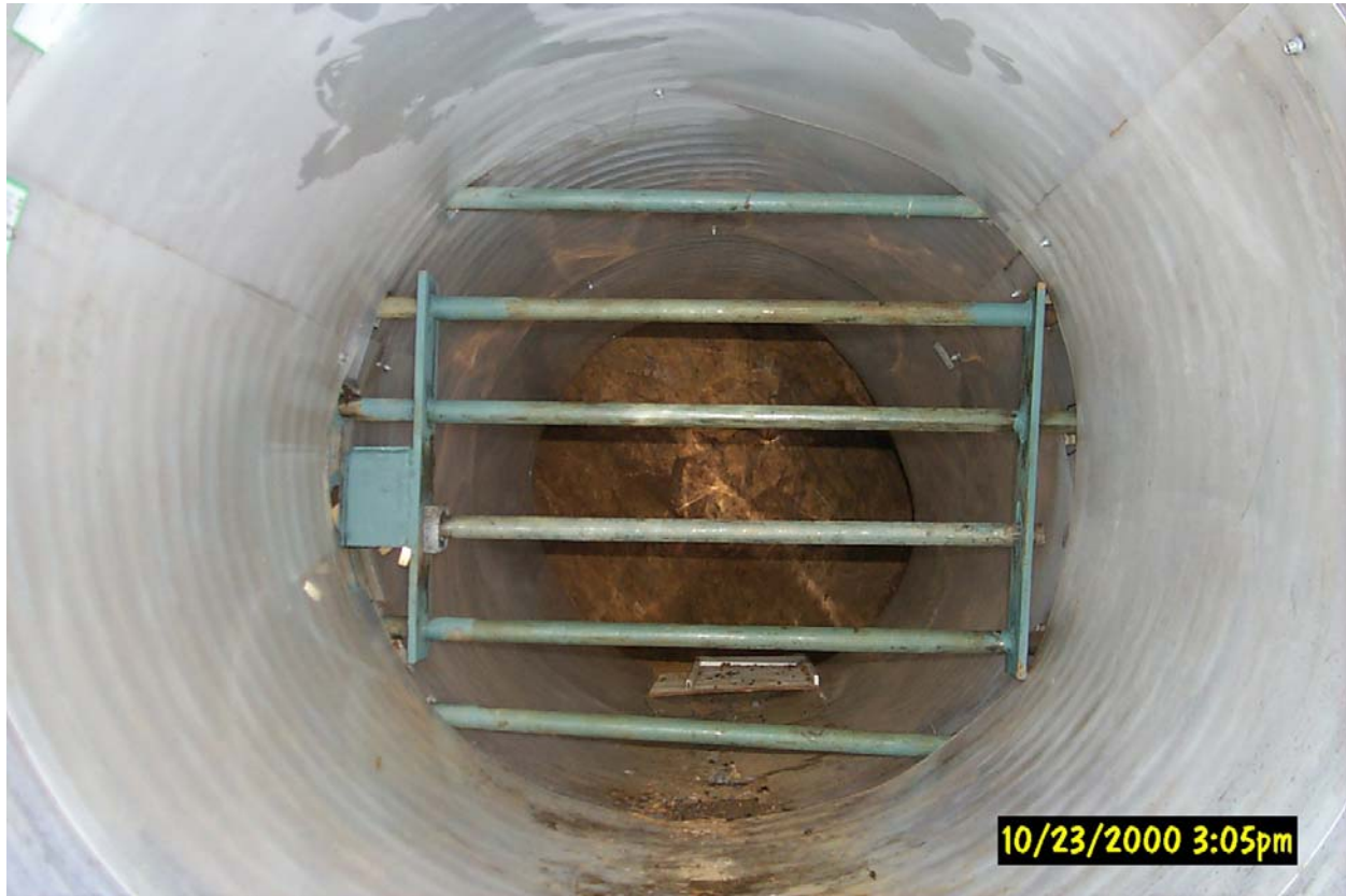
Photo 2: Example Bat Friendly Adit Closure with Access
