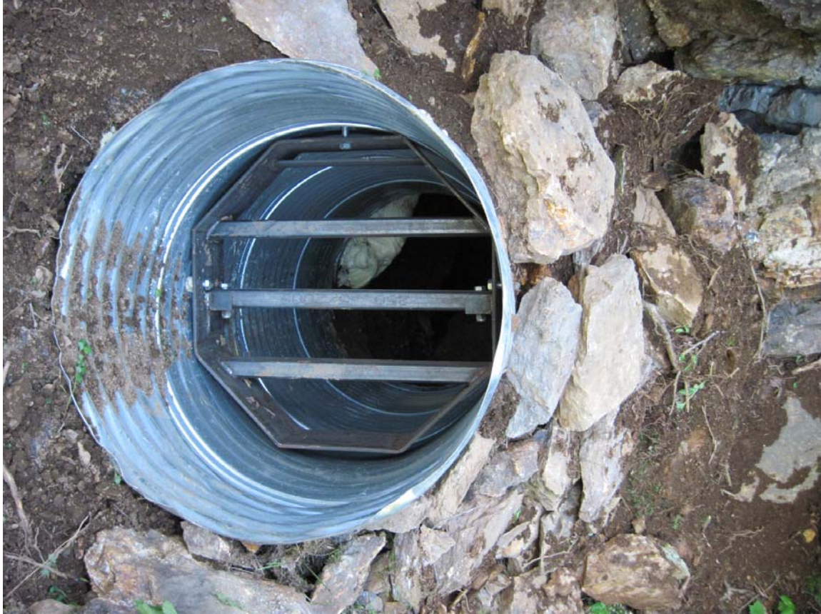
Photo 3: Example Bat Friendly Adit Closure with Access
