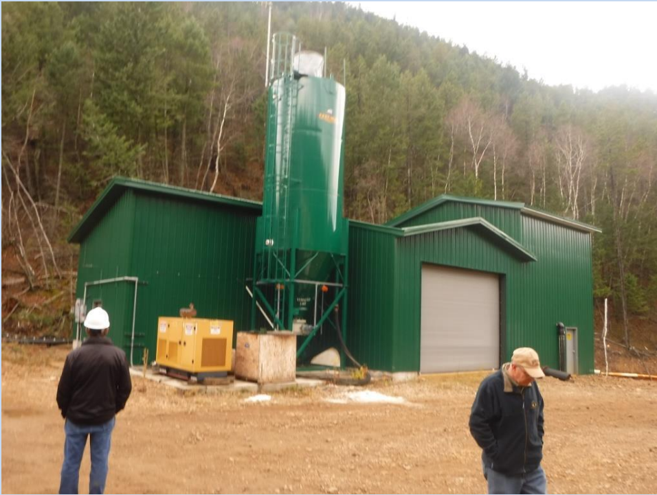
Zortman-Landusky Swift Gulch Treatment Facility
