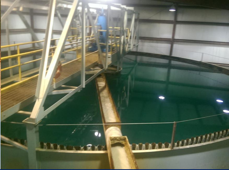
Landusky Treatment Facility
