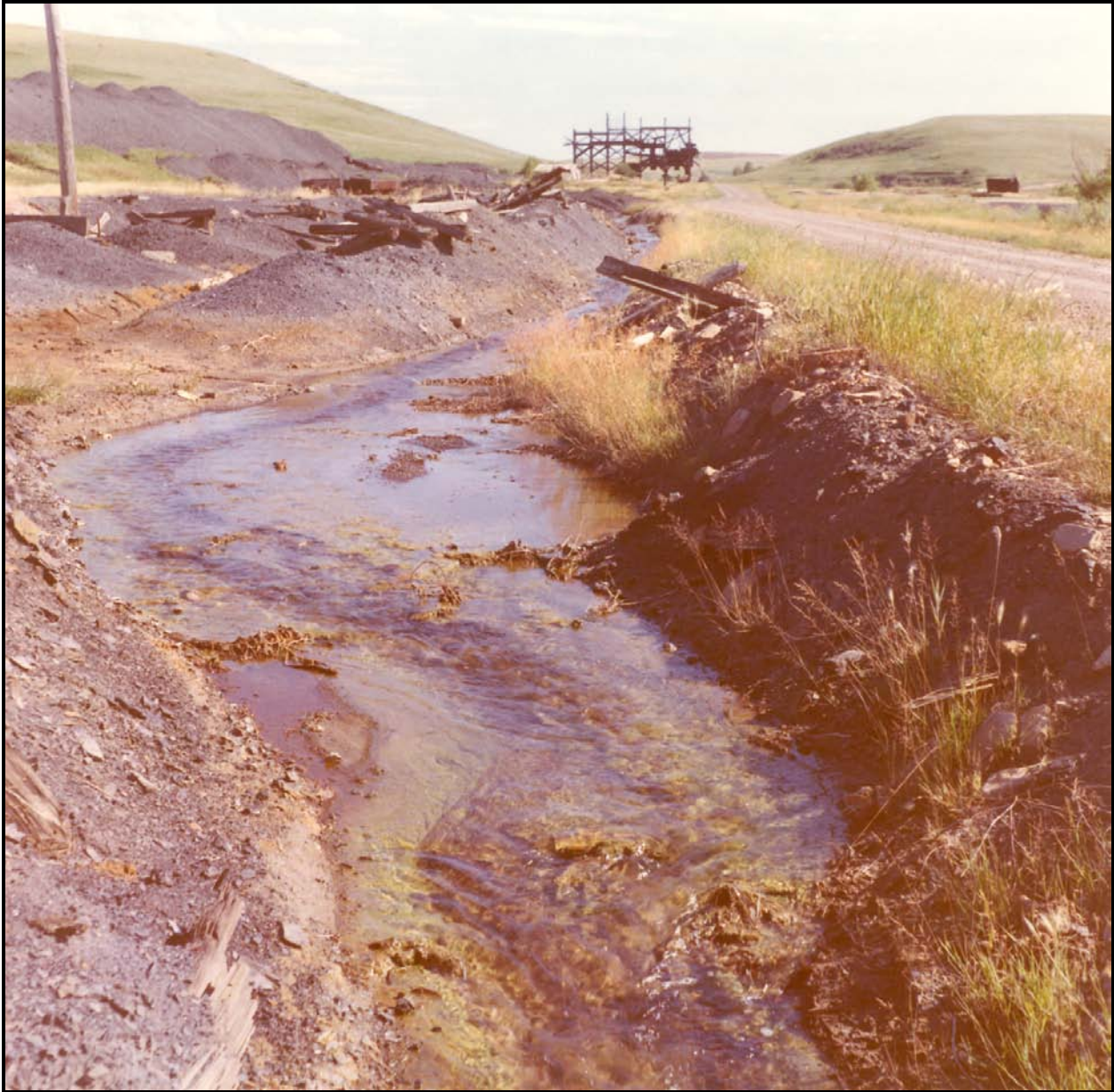
Figure 30. 1970 photograph of acid mine drainage at Giffen Mine (courtesy of Mine Waste Cleanup Bureau, Montana Department of Environmental Quality, Helena).
