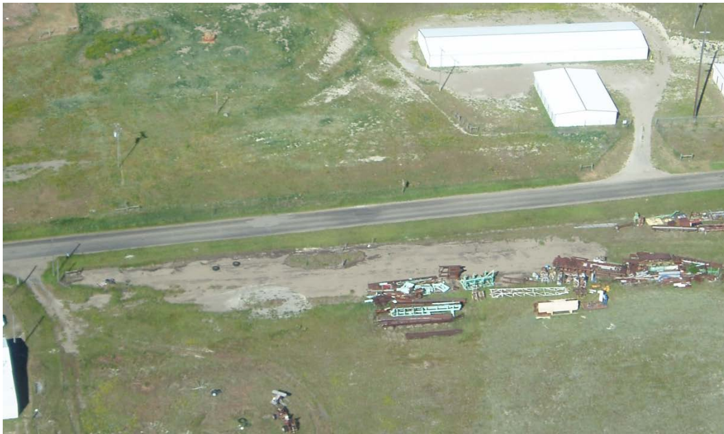
Figure 3. Aerial view of the Horsethief Road subsidence and grouting area. The in-road subsidence is the lighter area just left of center. The grouting area is the bare dirt stretch along the lower edge of the roadway.
