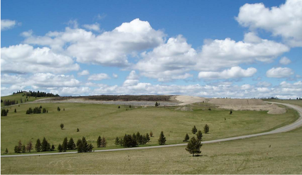
Figure 1. Overview of the Bald Butte repository
