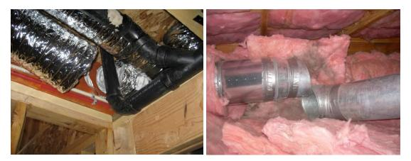
Duct tightness testing will identify significant duct problems such as disconnected duct joints. This is one reason why duct tightness testing is good practice even when all of the ducts are located within the building thermal envelope.
