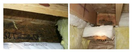
**Mold in Walls.** Both photos show mold behind unsealed electrical boxes. The energy code Air Barrier and Insulation Installation Table details code-required air barrier practices that would have prevented this problem from occurring. Because localized air leakage problems can occur, both the Air Barrier and Insulation Installation Table and building tightness testing is required by the energy code.
